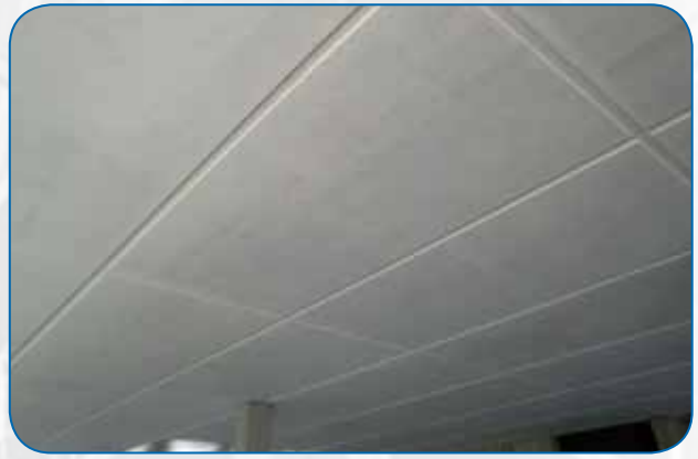
A fair faced exposed PT slab soffit. Photo: supplied by PTA.
