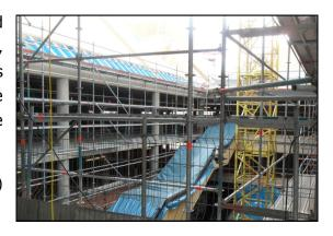
In line with the carbon neutral aspirations of the library, the thermal mass properties of the concrete were maximised by maintaining fair faced soffits, which will be finished with a wash to maintain the characteristic appearance of the concrete.
