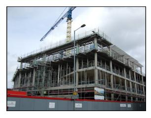
The building was originally schemed as a steel frame with precast units. However this could not satisfy the required floor zone restriction. It was then re-designed with traditional reinforced concrete floors, the slabs of which were of varying depths, typically 300mm, but with some areas of 400mm and 500mm.
