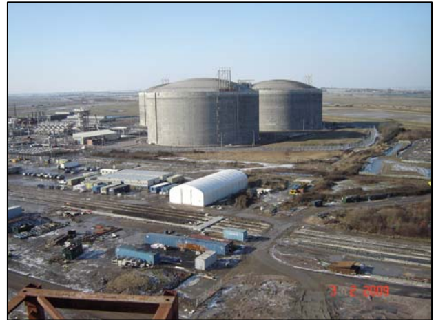
Overview of Tanks 1, 2 & 3
