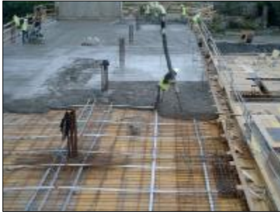
A floor slab being cast
