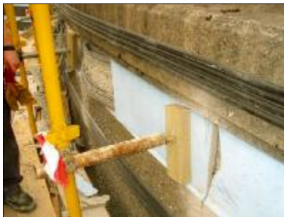
The live tanks needed temporary tendons
