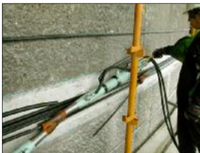
Checking jack extension during stressing
