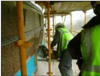
Strand cutting was carefully controlled
