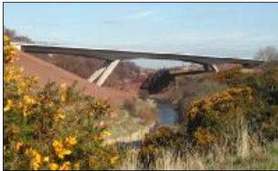
The bridge sits in a beautiful location
