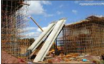
Major temporary works were required
