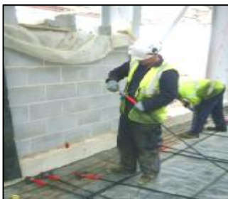
Dead anchorage installation
