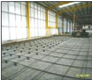
Conventional rebar reduced
