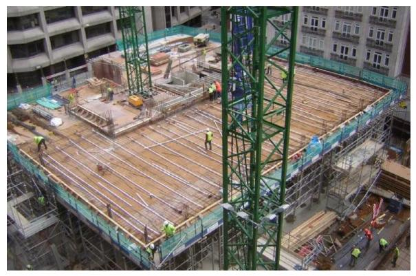
The post tensioning system allows for thinner slabs and larger floor spans...
