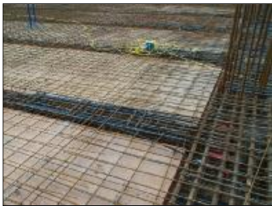
Dead end anchorage detail
