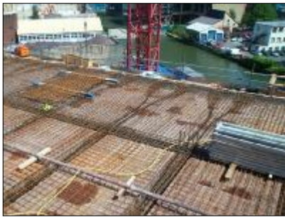
Slab detail showing long and short beams
