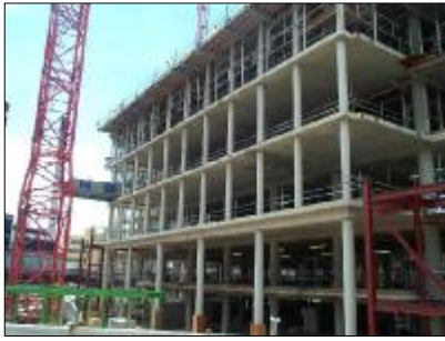
View on one wing of the building
