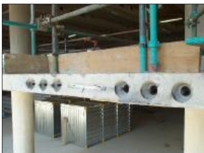
Anchorage pockets ready for filling
