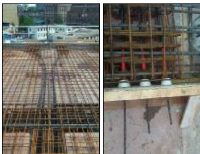
Unbonded tendons splay at the live end
