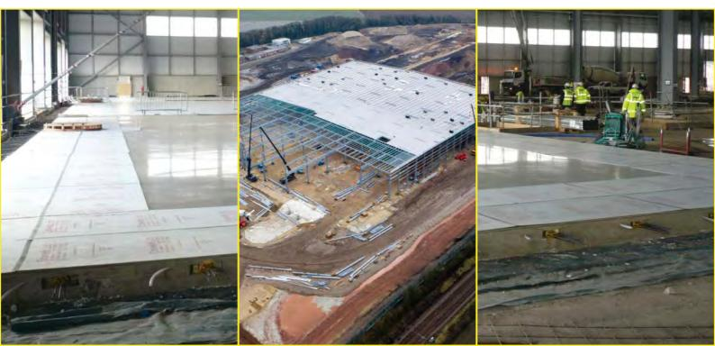
Critical in above assessment is the geotechnical properties of the sub grade, more so the sub grade modulus, which determines the spring support stiffness to the ground slab.
