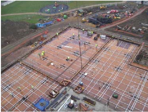
Podium slabs at North West level 1
