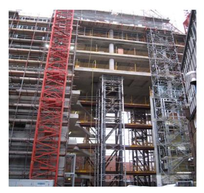
The heavy-lifting contract involved the transfer of 4 levels of insitu concrete structure over an atrium onto 2 spanning steel trusses by suspending the floors from 6 number 50mm Macalloy bars. Incremental loads were applied by 6 number 150T hollow ram jacks simultaneously through single control system. The key challenge was to monitor multiple systems employed to measure loads induced in jacks & 'lift-off' (load-deflection plot).
