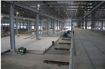
Original proposed RC solution was a 300mm thick slab but by using post-tensioning and benefitting from the improved load distribution and performance of a PT slab, this thickness was reduced to 180mm. Being a production facility the slab (approx grid size 150m x 165m) had to be designed to accommodate:
