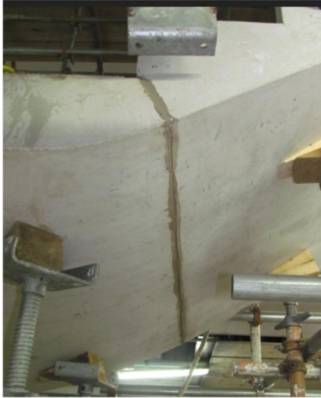
Fig. 06: Gaps between the Units Were Grouted
