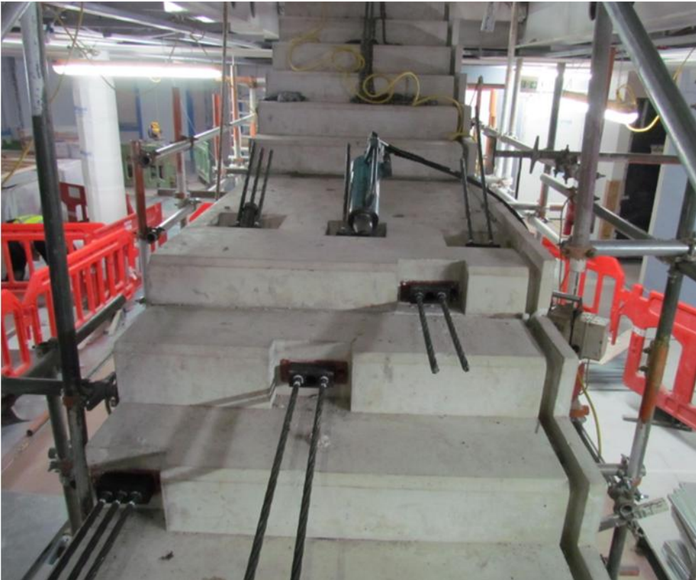
Fig. 04: Tendons Stressing at the Transition Location
