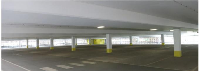
CCL was engaged to design, supply and install three levels of suspended post-tensioned beam and slab car park decks for the multi-storey car park constructed as part of the redevelopment of Ebbw Vale. The company was asked to provide a solution which would minimise the size and number of columns, eliminating intermediate columns in parking bays through a 16 m x 17.5 m grid, while at the same time providing a high degree of crack and deflection control.
